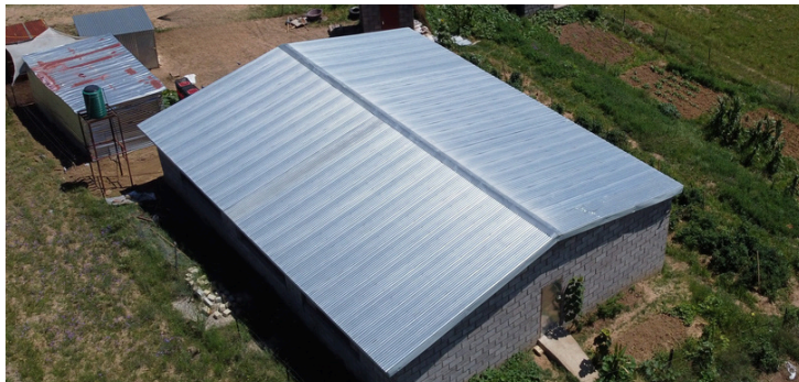
PHOTO 2.5 Corrugated Iron Roof Example
