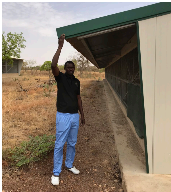
Pictures: Showing overhangs for water runoff and providing shade Courtesy of Hendrix Genetics
